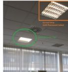
B4 – Office area
